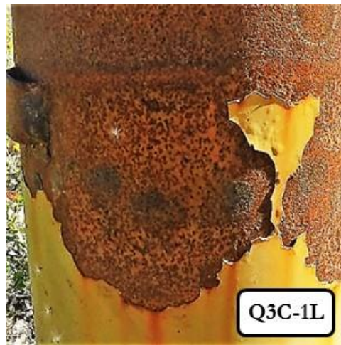
Figure 3.9 Severely delaminated coating line accompanied by widespread pack rust and pack out on ladder clip.
