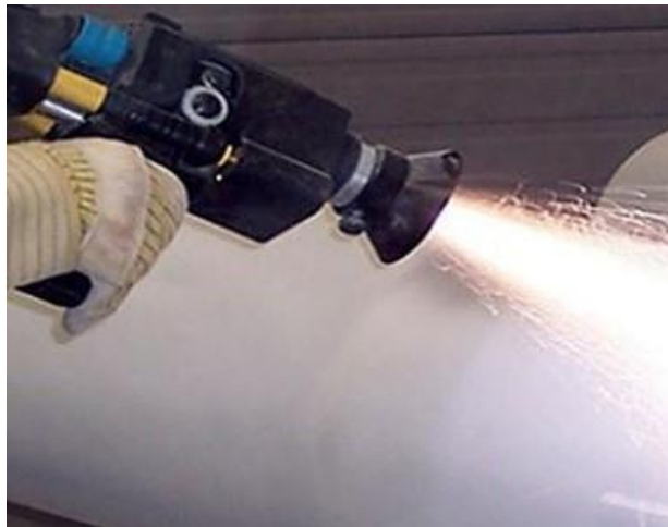
Figure 7.1 Metallizing of steel pole.
