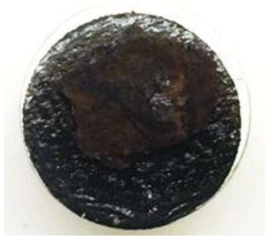
Figure A.3 Pack-rust sample from coating line region of Pole Q3C-2L at Site 2.
