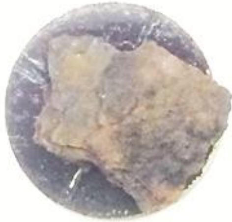
Figure A.13 Loose rust sample from GS fastener region of Pole 8Z-2R at Site 5.
